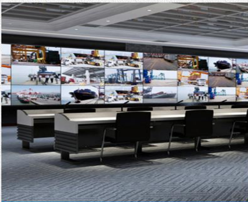
Large computer room
