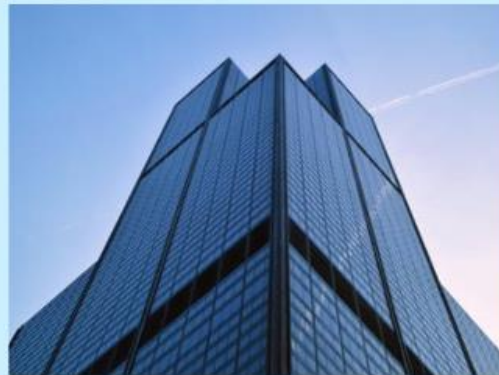
Smart building cabling
